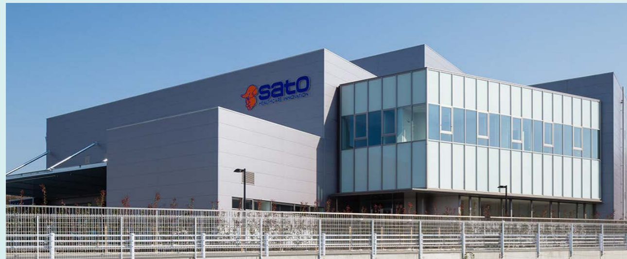
Tokyo Distribution Center
