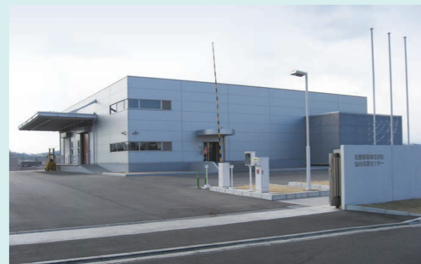
Sendai Distribution Center
